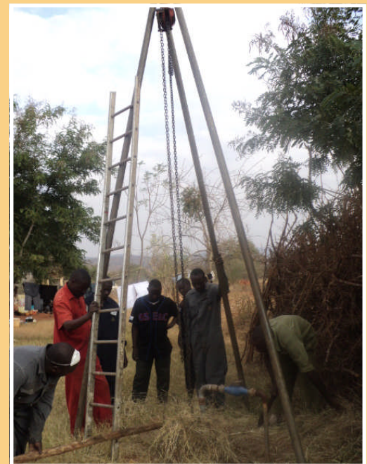
Pulling up the water pump
